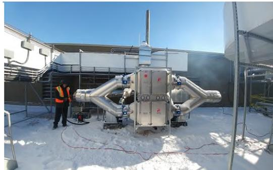
*Redundant B2-series (separate pre-filter door) BIBO on AIR exhaust application. Stacked filter arrangement with duct manifold in and duct manifold out to redundant fans.*
