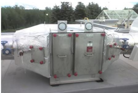
Condensation is going to be a problem for any Bag-in/Bag-out (BIBO) Filter equipment located outdoors, particularly in lower temperatures and in colder climates. Warm and humid building air will migrate upwards (even when the fans are off) through the exhaust duct and into the steel filter box where it will condense out when it hits the cold stainless-steel.
