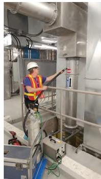
Step 4) After testing is completed ensure the port is plugged (or capped) to eliminate air leakage (*lower right*).
