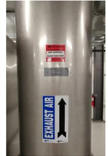
Step 3) Start the exhaust fan(s) and take flow measurements to ensure there is adequate draw to pull the challenge aerosol into the filters being challenged. Accredited technician injects the challenge aerosol into the preselected injection port, note that the port should be at an easily accessible location whenever possible (*lower right*).
