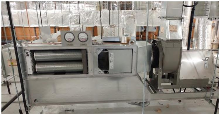
**Filter-Fan Units** can be packaged with any in-line filter housing. HEPA/ULPA filter housings can be mated to utility fans and they can also be put into series with other filter housings including carbon-tray or carbon-canister housings to address both chemical/odor and particulate capture.
